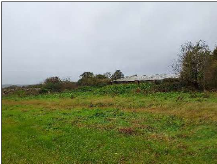
Figure 5. Tree groups and scrub vegetation around derelict dwelling and barn in centre of site.
