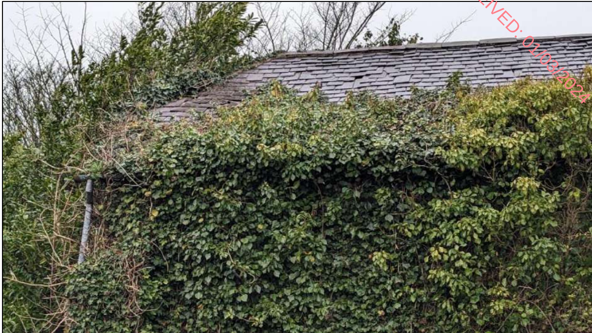
Plate 3-2: Building on-site with features suitable for roosting bats
